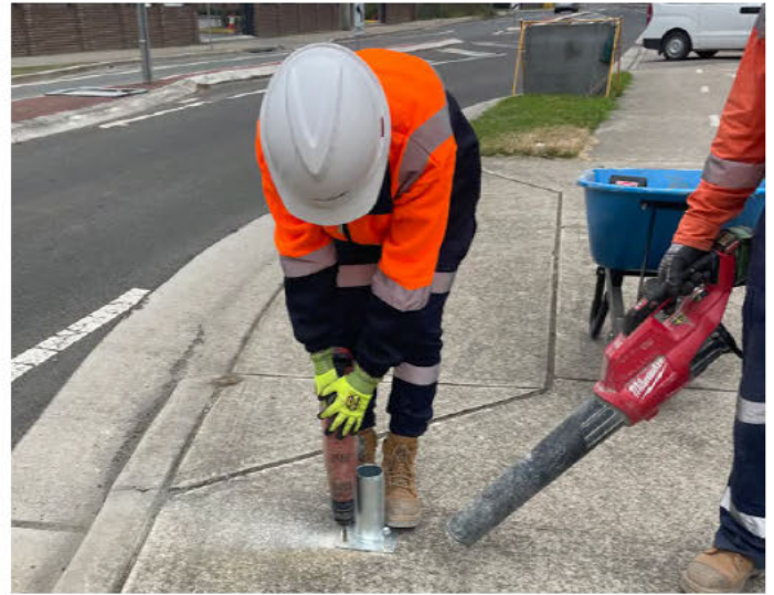
Figure 22: School based trainee installing sign mount
