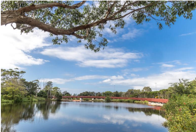
Photo: Bridge over Scarborough Park ponds
