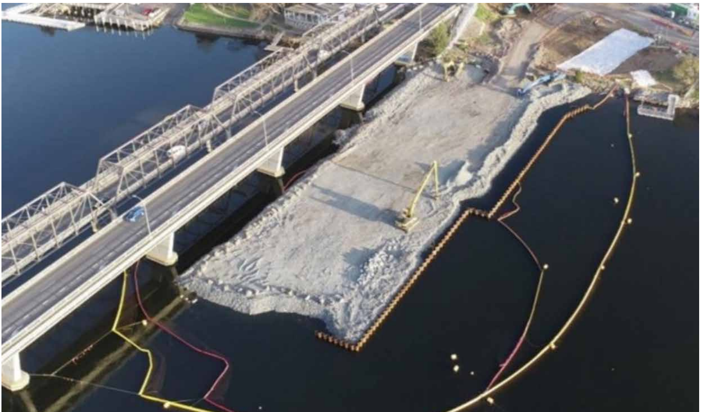
Example of rock platform construction (Nowra Bridge)
