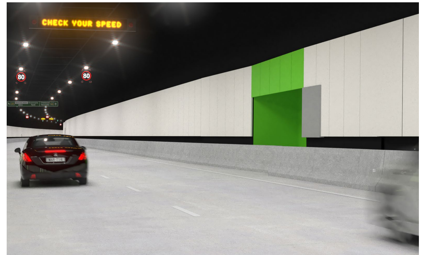
Artist's impression: Typical emergency cross passage to provide safe and legible egress
