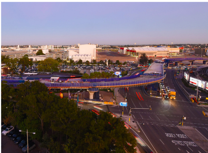
Work continuing on the Departures ramp over Sir Reginald Ansett Drive, Mascot.
