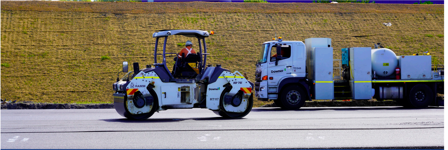
Asphalting work has begun on the Project.
