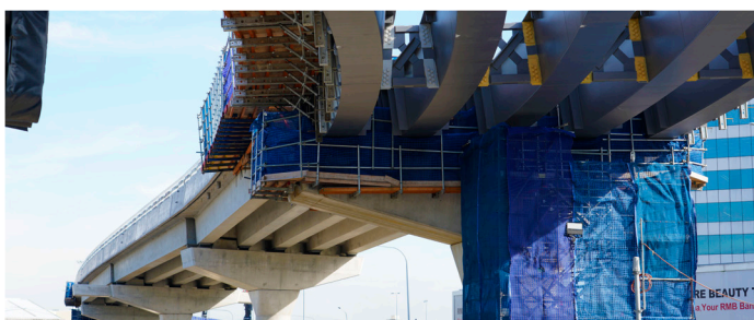
Continuing girder installation on Qantas Drive, Mascot.
