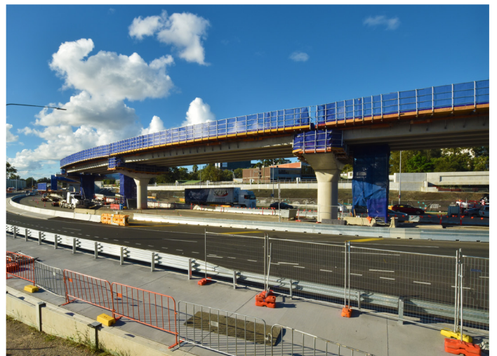
Girder installation on Qantas Drive, Mascot.
