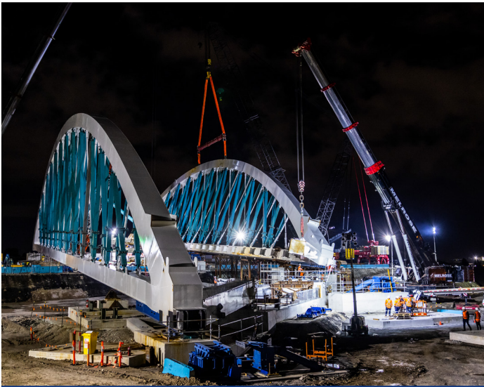
Workers assembling the Twin Arch Bridges at Tempe.
