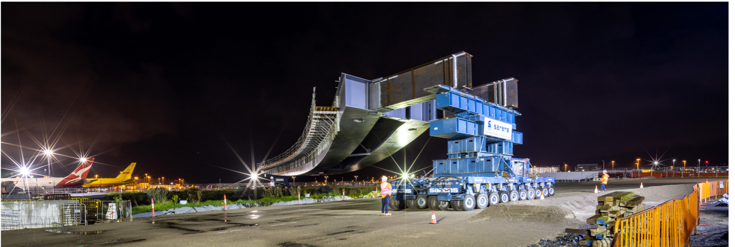
Ongoing bridge construction in St Peters.
