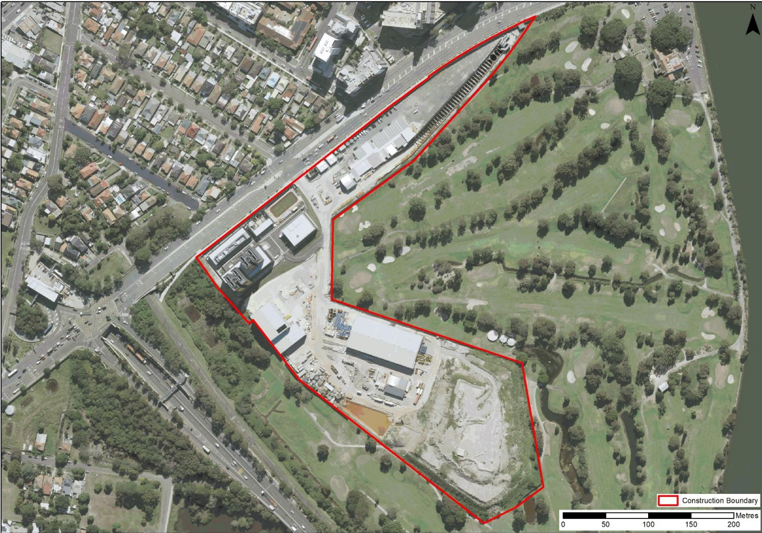
Figure 1.2: Existing site compound at Arncliffe. Image provided by CGU.
