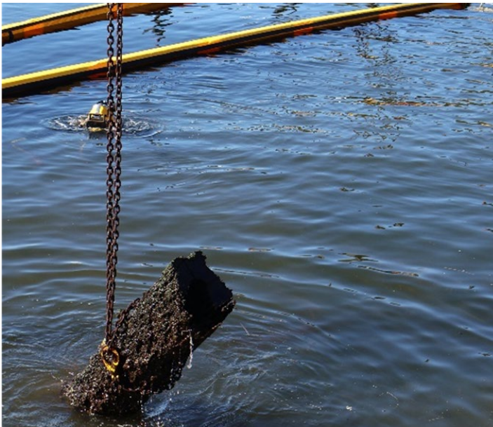
Derelict marine infrastructure removal work underway (foreground) with diver (background).
