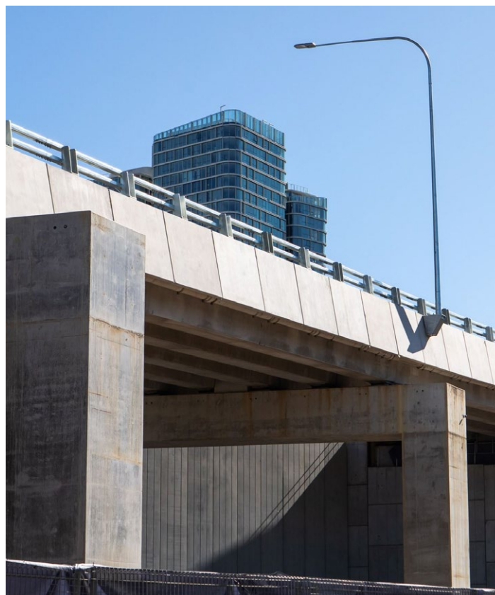
Alfred Street off ramp viewed from Alfred Street North.
