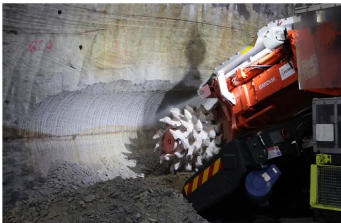
Western Harbour Tunnel roadheader excavating material that will be repurposed in other locations.
