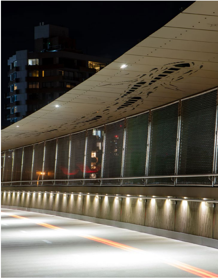
Falcon Street shared user bridge at night.
