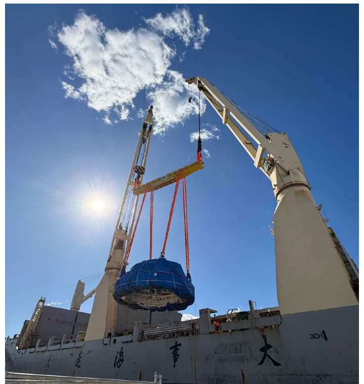
Unloading the 325 tonne 'main drive' component of our TBM, Patyegarang, at Glebe Island.
