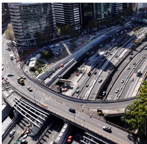
Image: High Street bridge widening and new northbound on ramp in March 2025.
