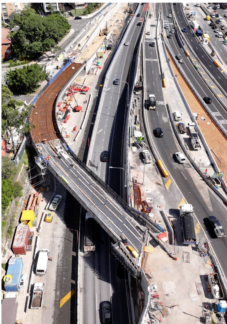
Image: Falcon Street southbound bus ramp in March 2025.
