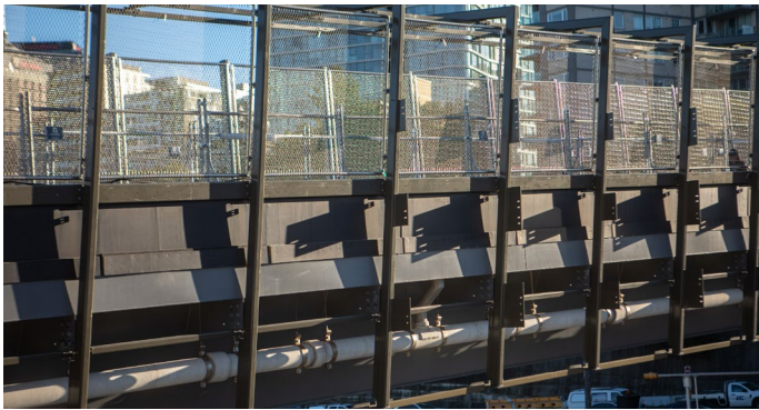
Image: Ridge Street shared user bridge in June 2025.
