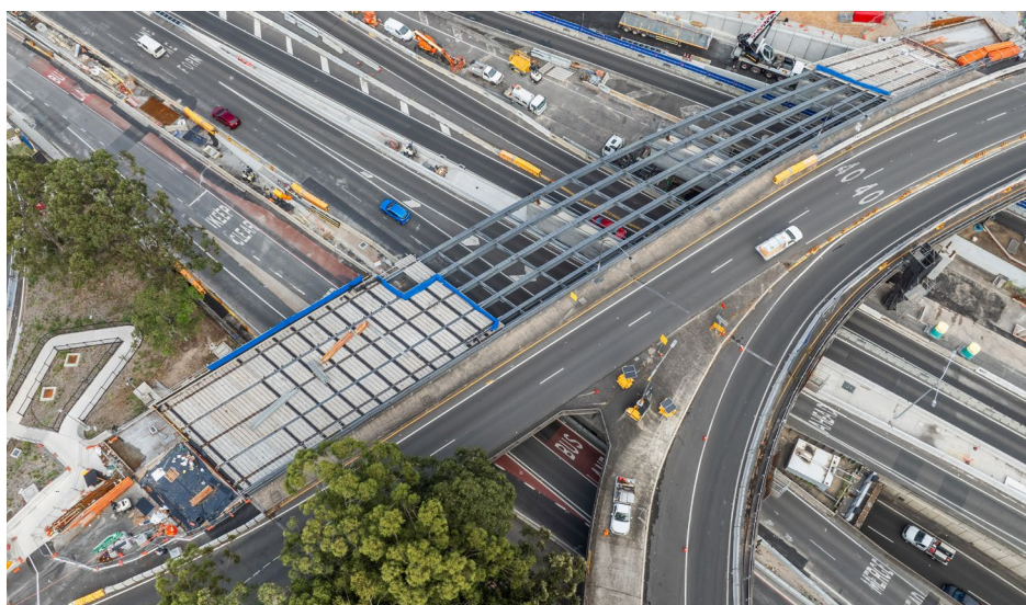
Image: High Street bridge widening in April 2025.
