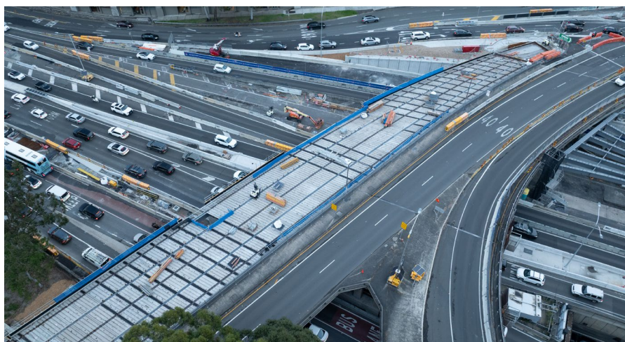
Image: High Street bridge widening in May 2025.
