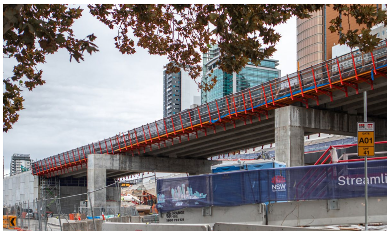
Image: Alfred Street off ramp in March 2025.
