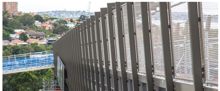
Image: Ridge Street shared user bridge in March 2025.
