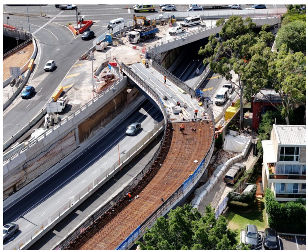
Image: Falcon Street southbound bus ramp in March 2025.
