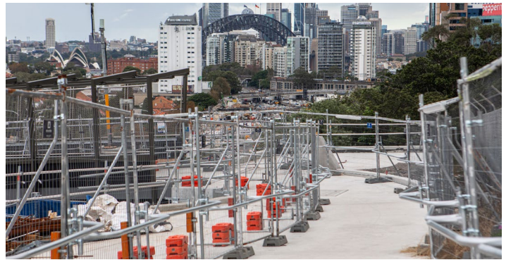
Image: Ridge Street shared user bridge in March 2025.
