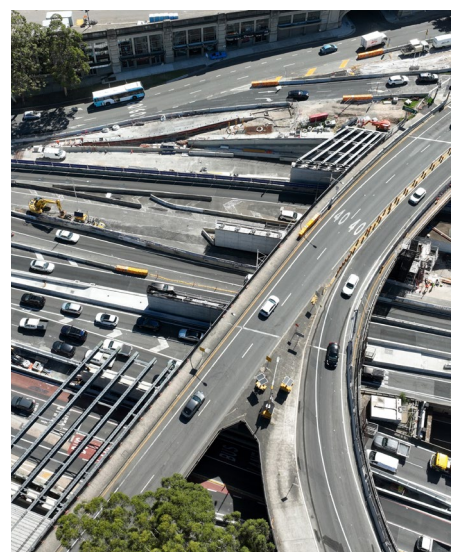
Image: High Street bridge widening in December 2024.
