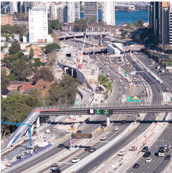
Image: Ridge Street shared user bridge in June 2025.
