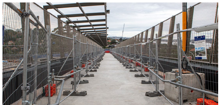
Image: Ridge Street shared user bridge in March 2025.
