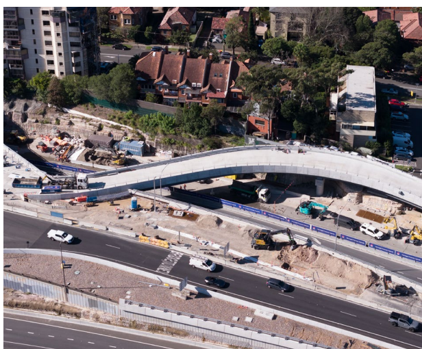
Image: Falcon Street southbound bus ramp in June 2025.
