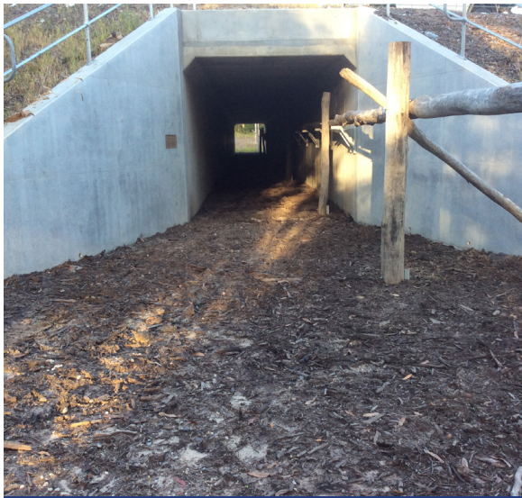
example of a fauna underpass
