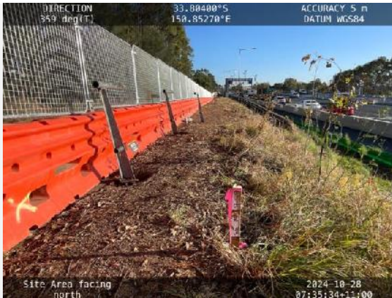
Photo 2: 28/10/2024: View from top of the embankment at the central portion of the site, facing north of M7 Motorway.
