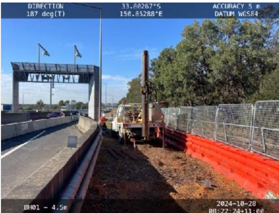
Photo 3: 28/10/2024: Photo taken north of BH01, facing south of M7 Motorway.
