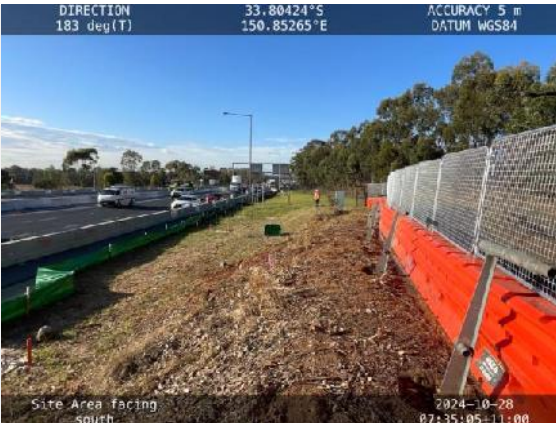
Photo 1: 28/10/2024: View from top of the embankment at the central portion of the site, facing south of M7 Motorway.
