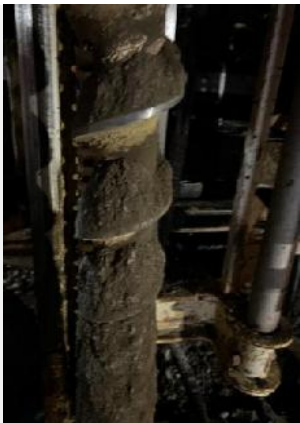
Photo 17: 20/11/2024: Photo of clayey silt fill at 0.5 mBGL of BH09
