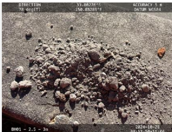
Photo 6: 28/10/2024: Photo of sandy clay fill at 2.5 mbgl of BH01
