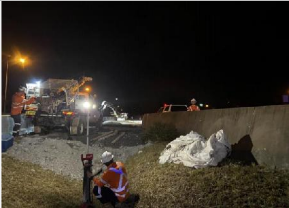
Photo 16: 20/11/2024: View of central and southern portion of median strip, showing backfilled area, facing south.
