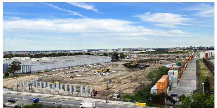
View from St Peters Interchange of our Northern Lands site.
