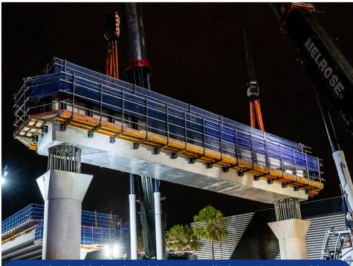
The double headstock being installed over Sir Reginald Ansett Drive, Mascot.
