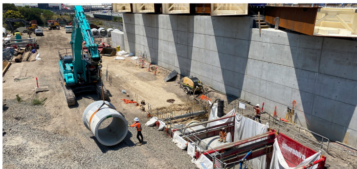
Drainage work during the holiday rail possession.
