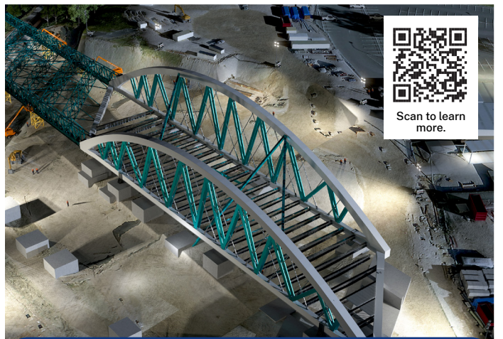
An artist's impression of the Twin Arch Bridge showing the arches with the teal coloured temporary struts.
