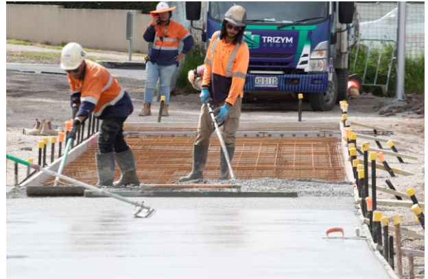
Image: Concreting work in progress, February 2025.
