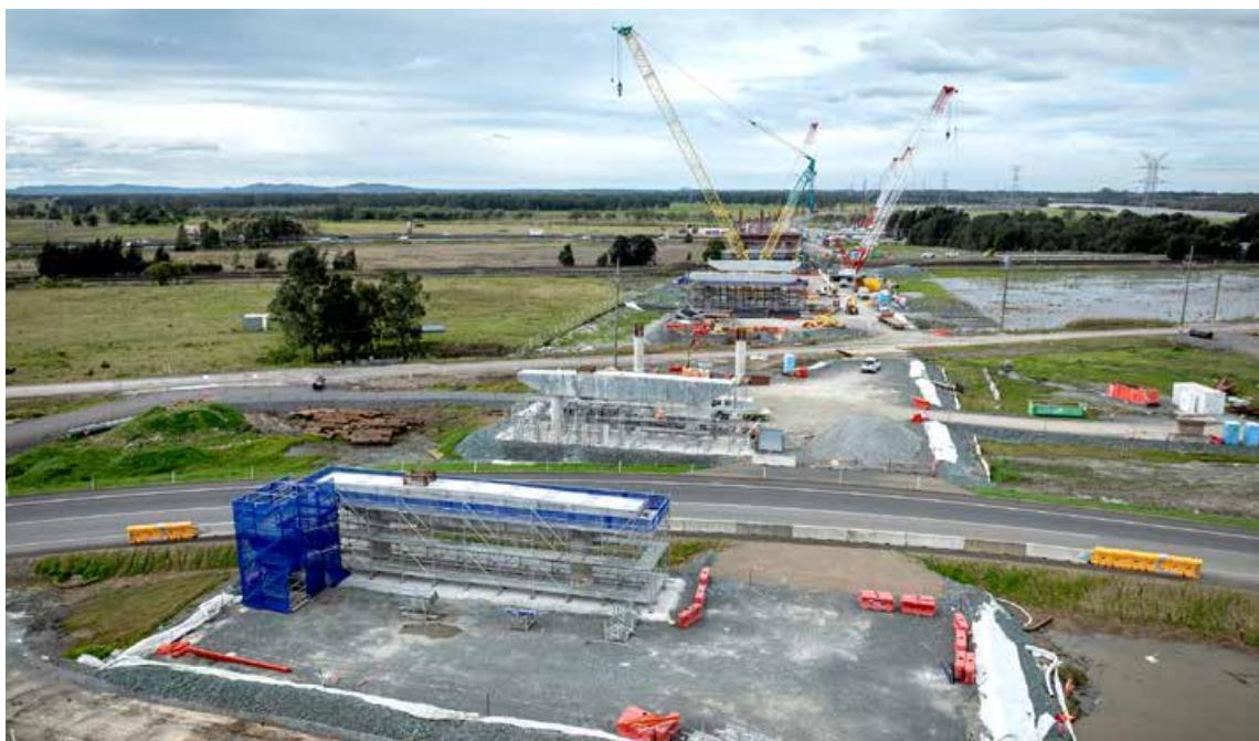
Figure 3.4 Construction of headstocks and columns for the viaduct at Tarro
