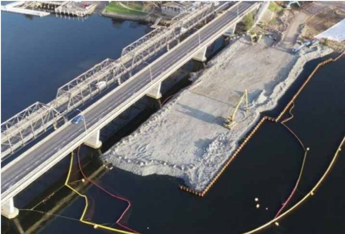
Figure 1.3 Example of rock platform construction (Nowra Bridge)
