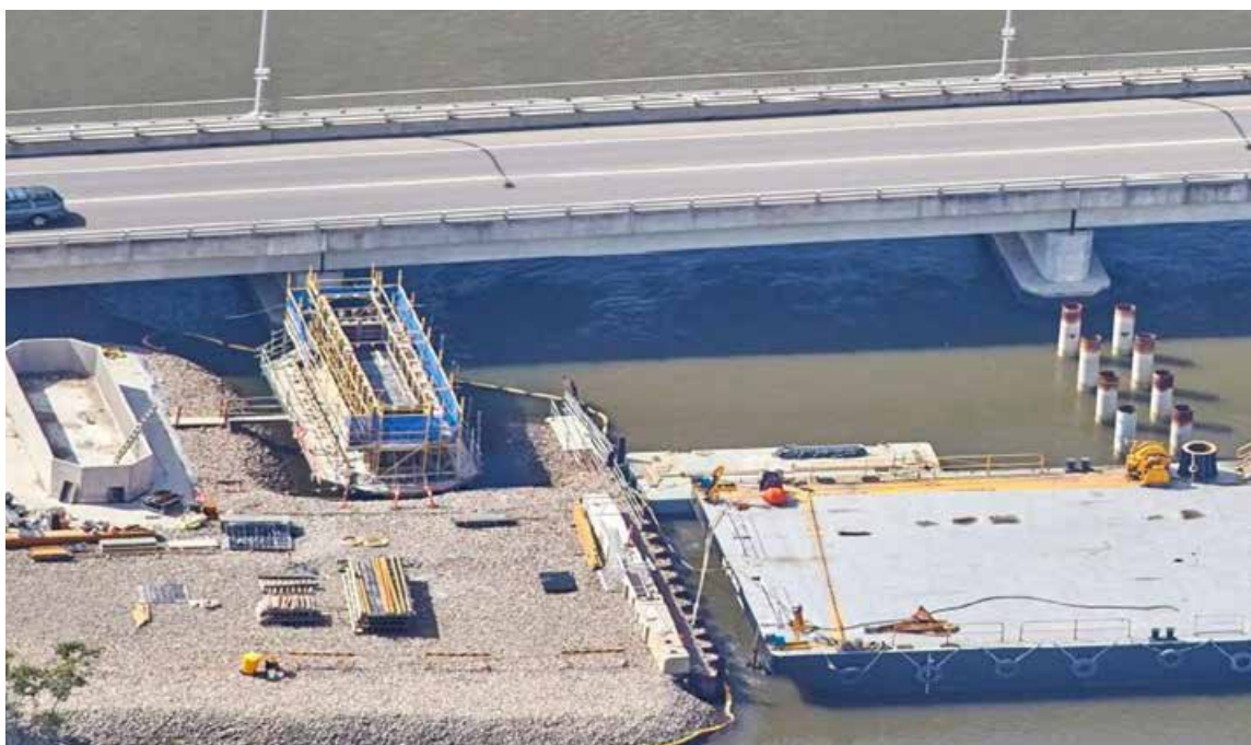
Figure 1.2 Example of barge-based construction – Tourle Street Bridge
