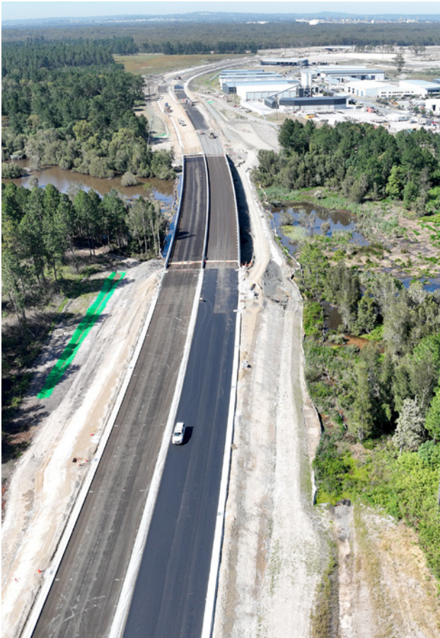
Windeyers Creek bridge preparation for asphaltting
