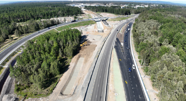
Water quality basin construction at the Raymond Terrace interchange
