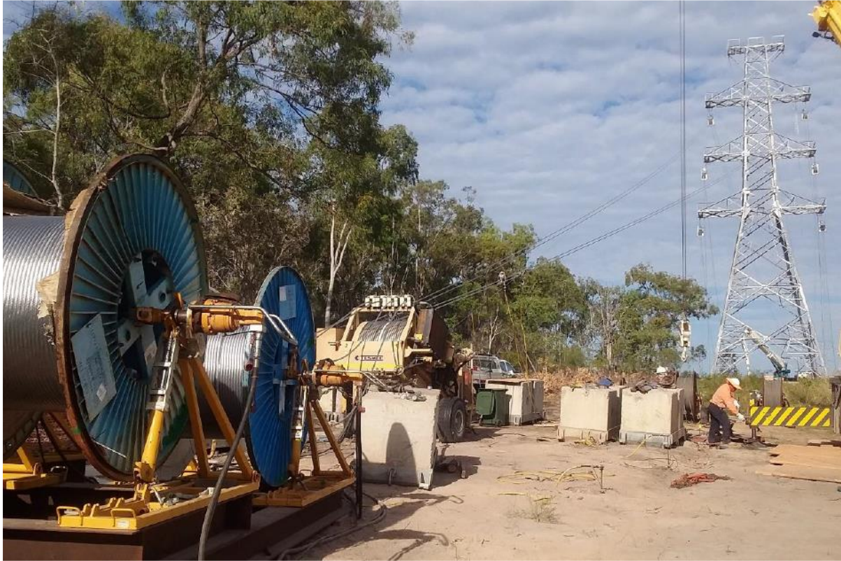
Plate 7-7: Brake site from where the conductor is pulled out under tension
