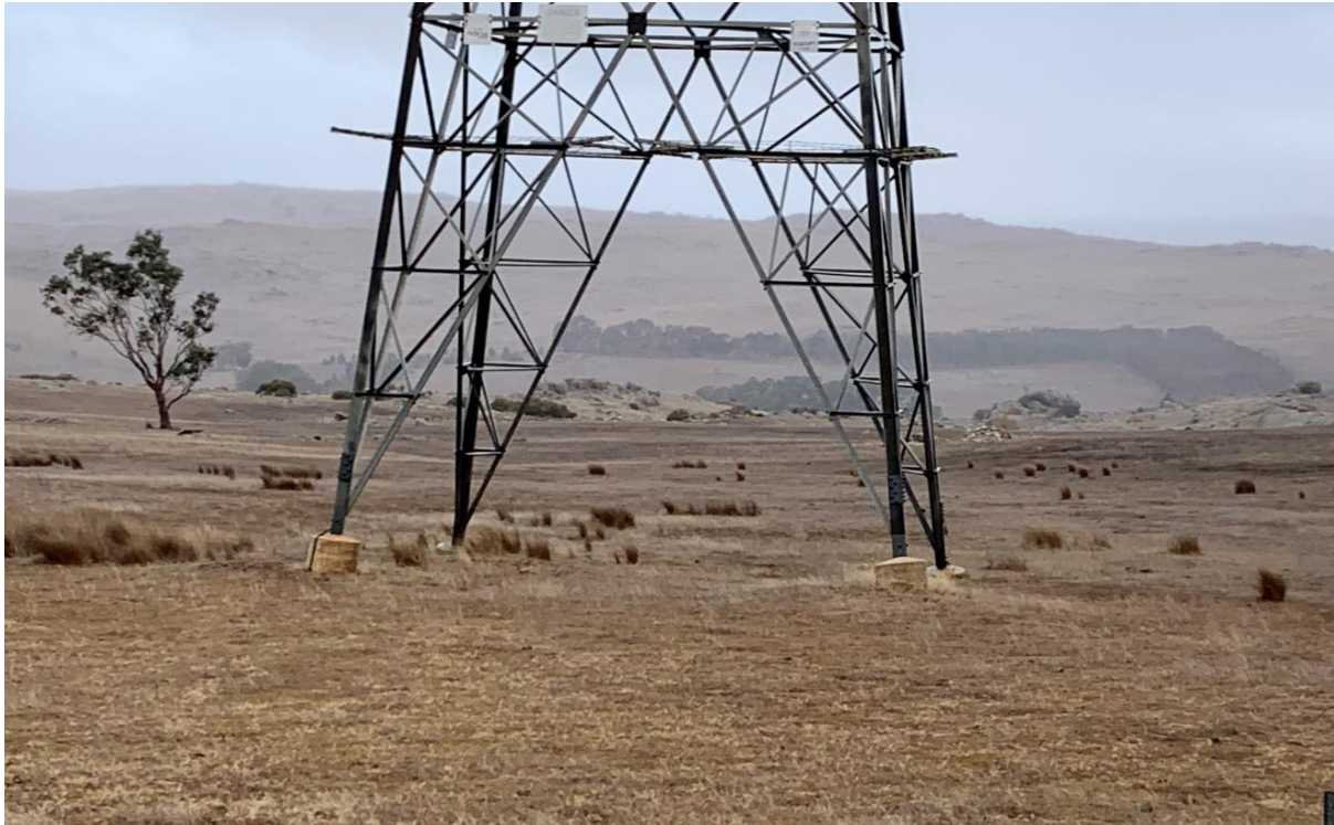
Plate 7-2: Base of typical lattice tower
