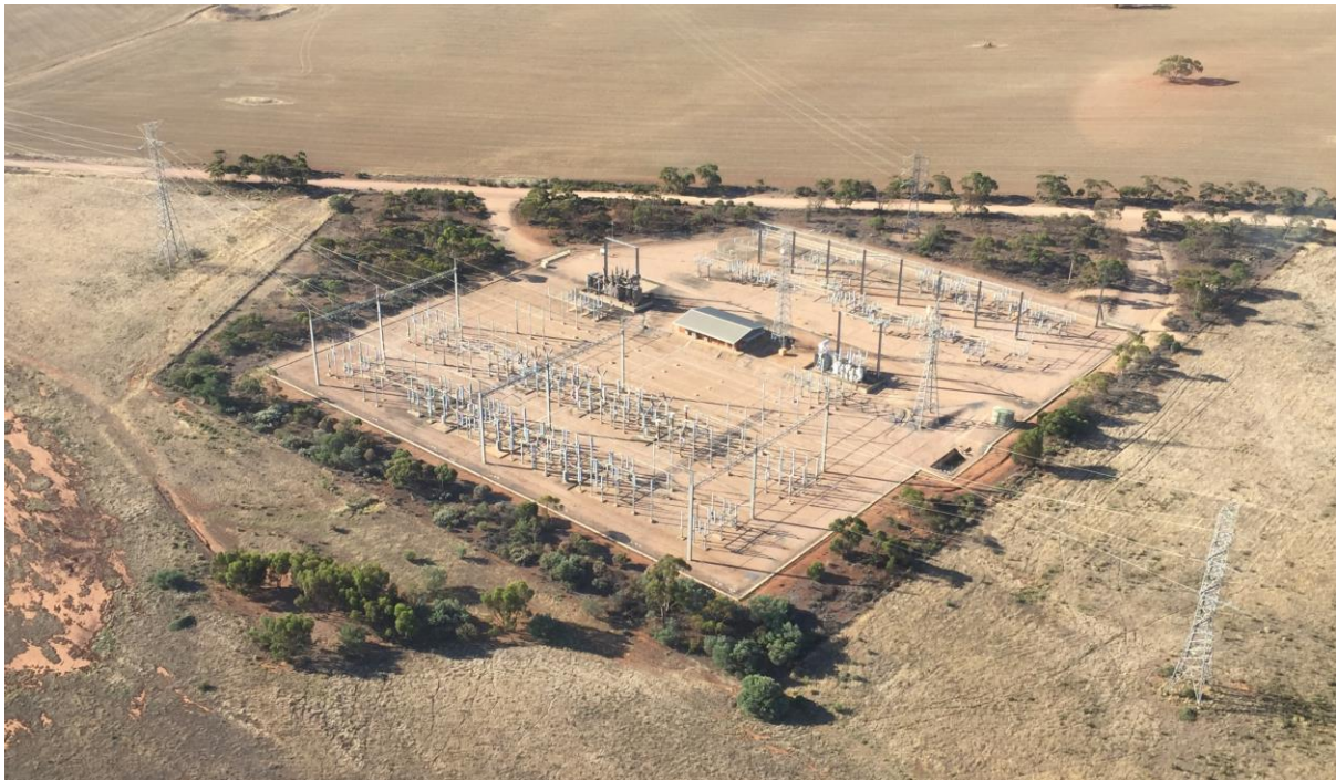
Plate 7-1: Existing Robertstown substation
