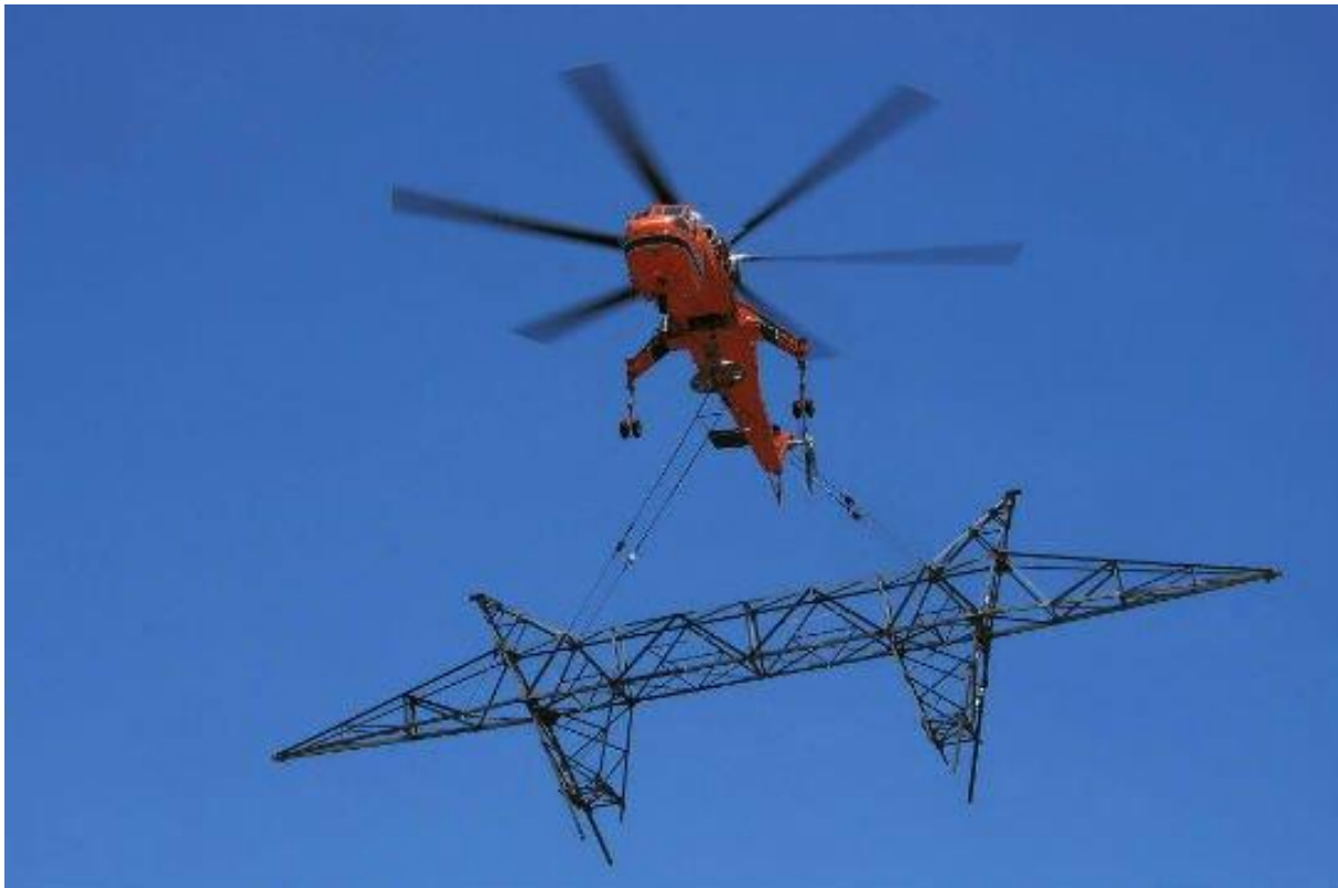
Plate 7-6: Examples of helicopter lifting and tower transport
