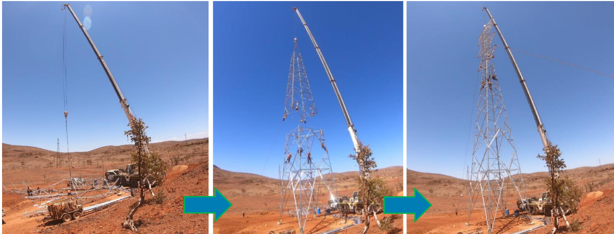
Plate 7-5: Example of tower assembly and erection
