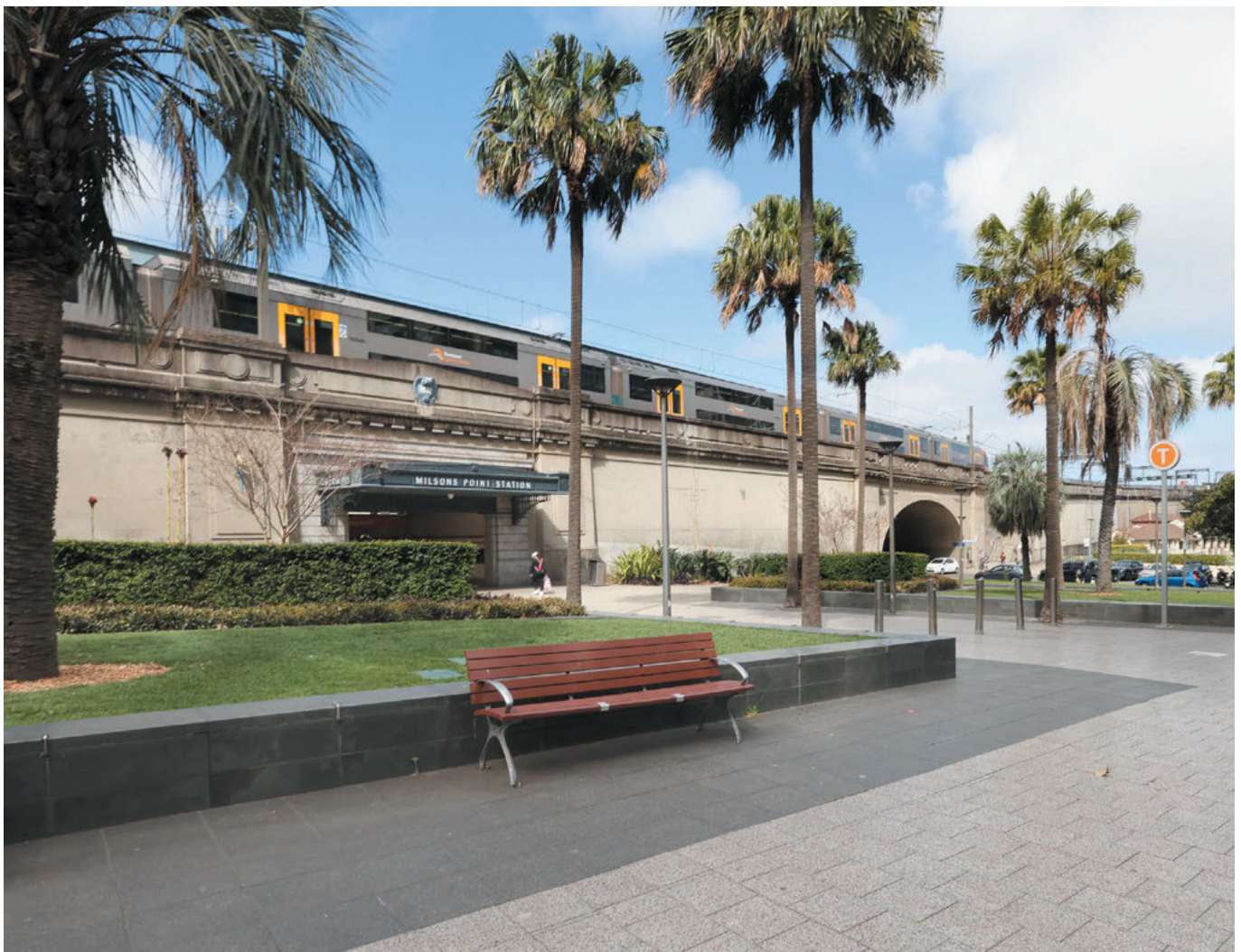
Milsons Point Station Plaza
