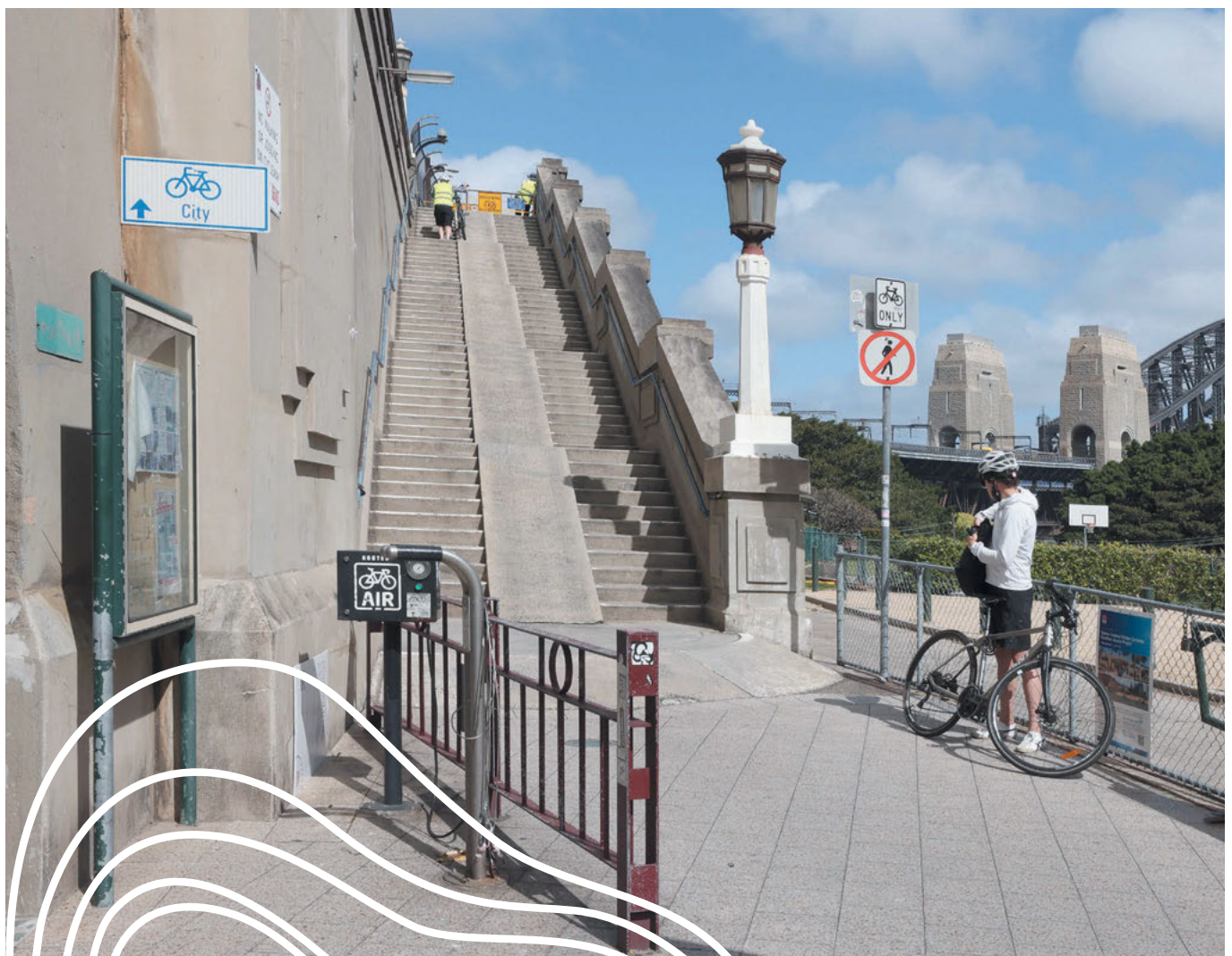
Steps to the Sydney Harbour Bridge Cycleway
