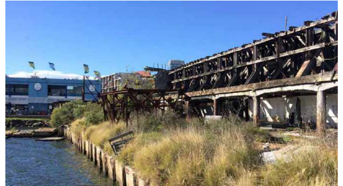
Rear view of existing coal bin loader looking east towards the existing Fish Market.
