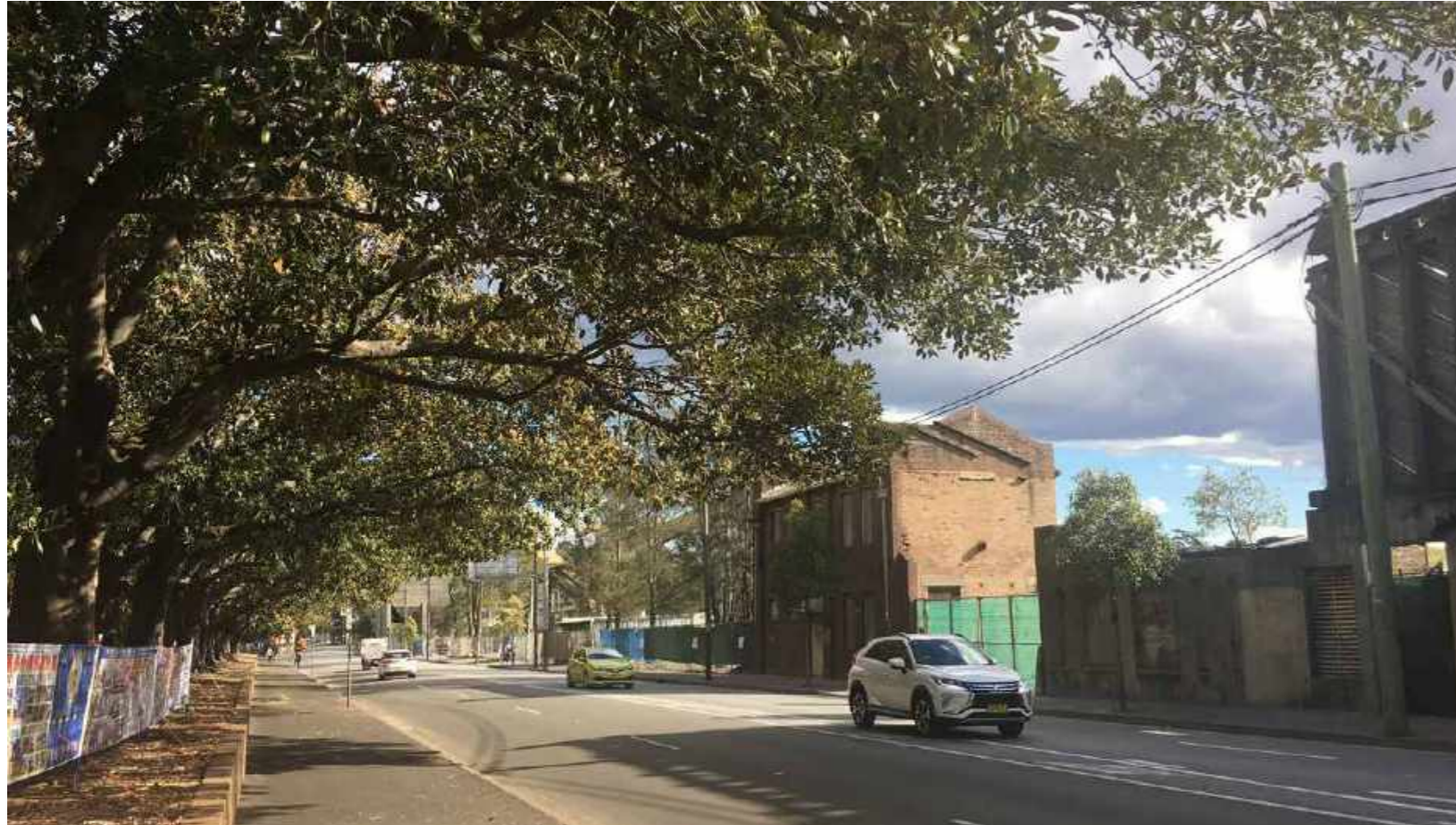
View of existing Bridge Road looking west from northern edge footpath of Wentworth Park. Existing brick building and coal bin loader on right.
