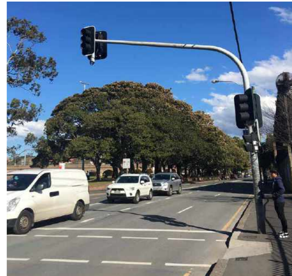
View to west from Bridge Road and Wattle Street traffic intersection.
