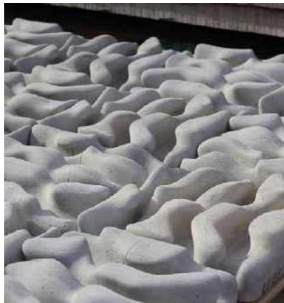
3D printed Seawall by Reef Design Lab before and after installation - Project by SIMS
