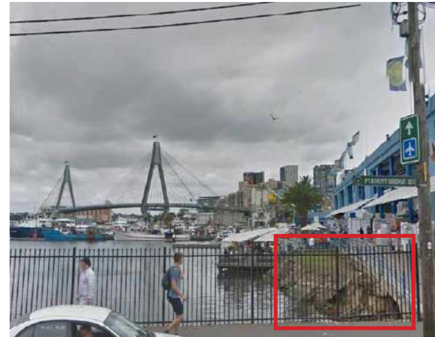
5. Remnant Sandstone Sea Walls
