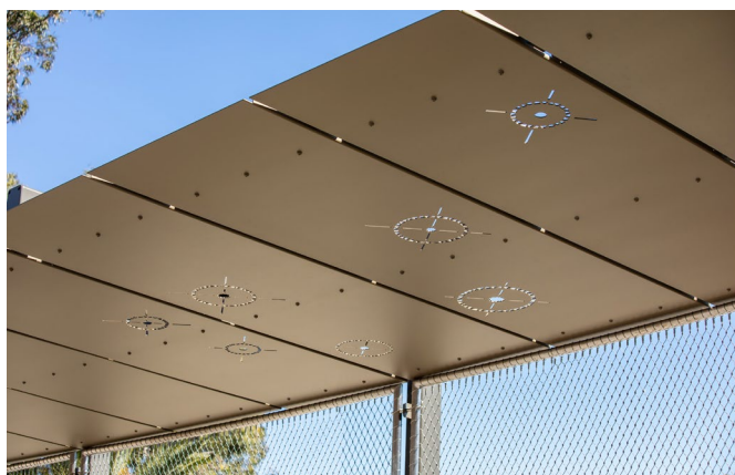
Picture 2: Falcon Street shared user bridge, shade canopy.
