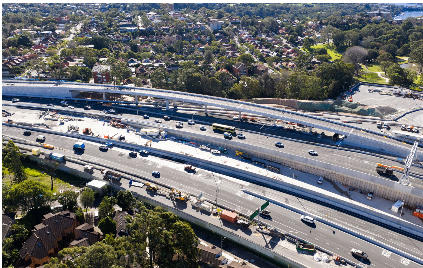
Picture 7: The Miller Street southbound on ramp, view east.
