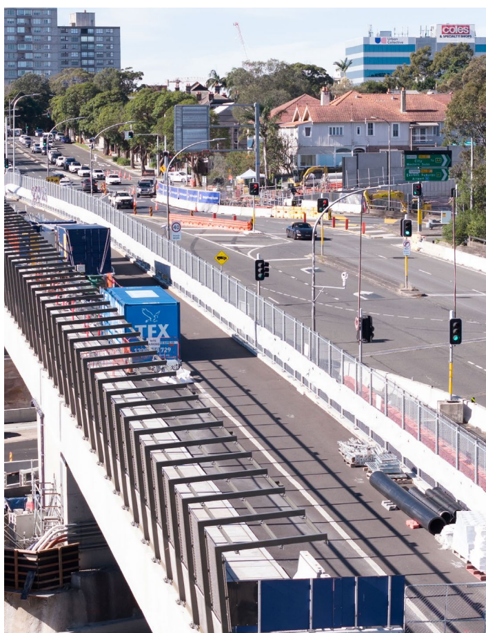
Picture 4: the new Ernest Street shared user bridge, view east on Ernest Street.
