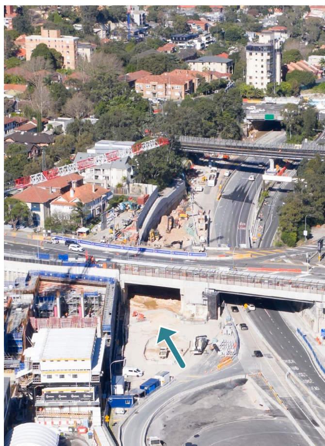
Picture 5: the new Ernest Street underpass, view of the southbound outer lanes.
