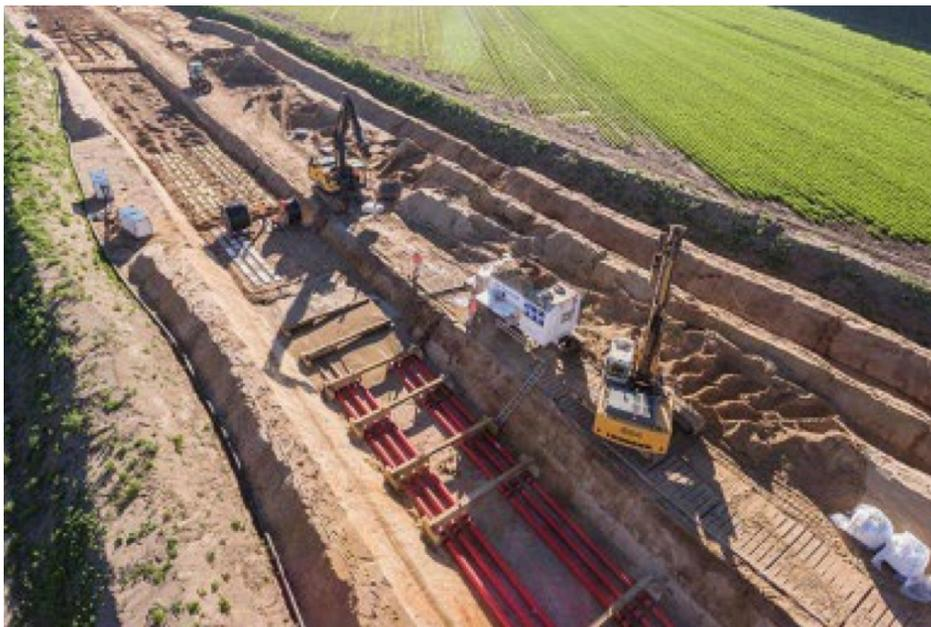
**Pictured:** Direct buried cable installation in a rural area. This buffer will run the entire length of the route.
