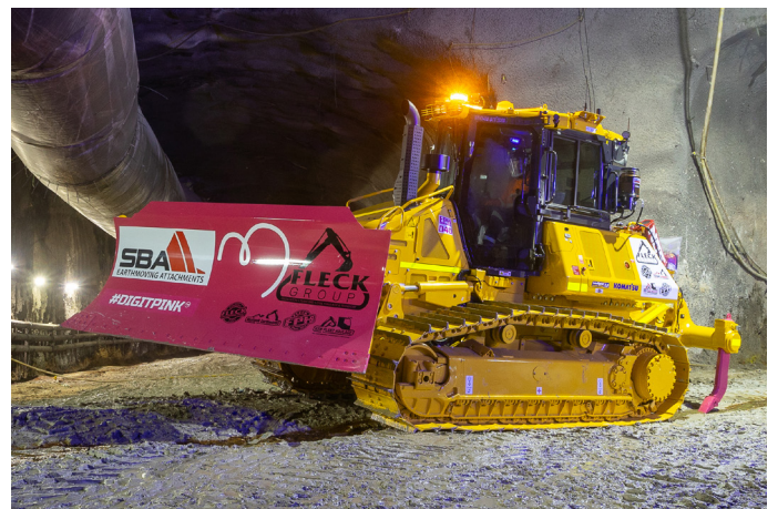
Dozer in the Arncliffe south shaft passage, November 2024
