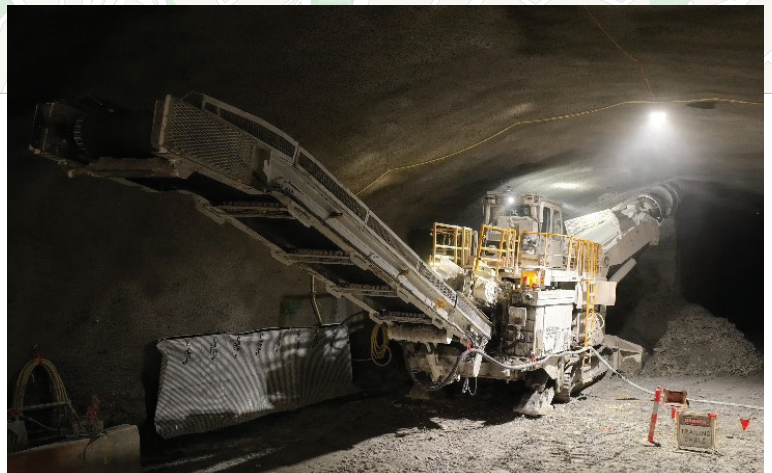
Roadheader in operation during underground excavation
