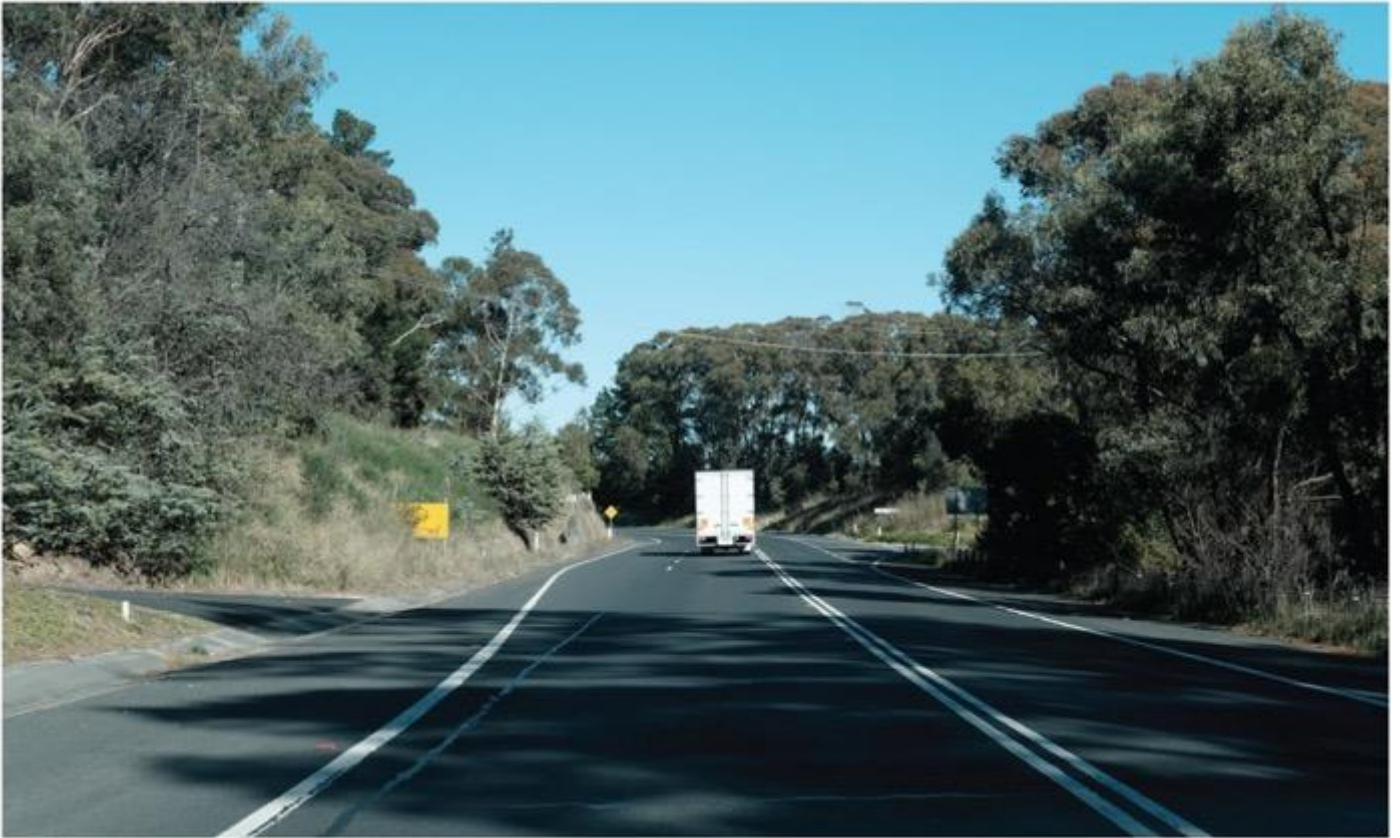
Figure 6-52 Viewpoint 25 (existing) from Great Western Highway, near the intersection of Old Bathurst Road, looking south.
