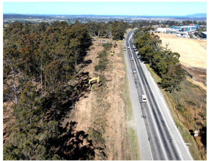
Clearing at the Northern Connection
