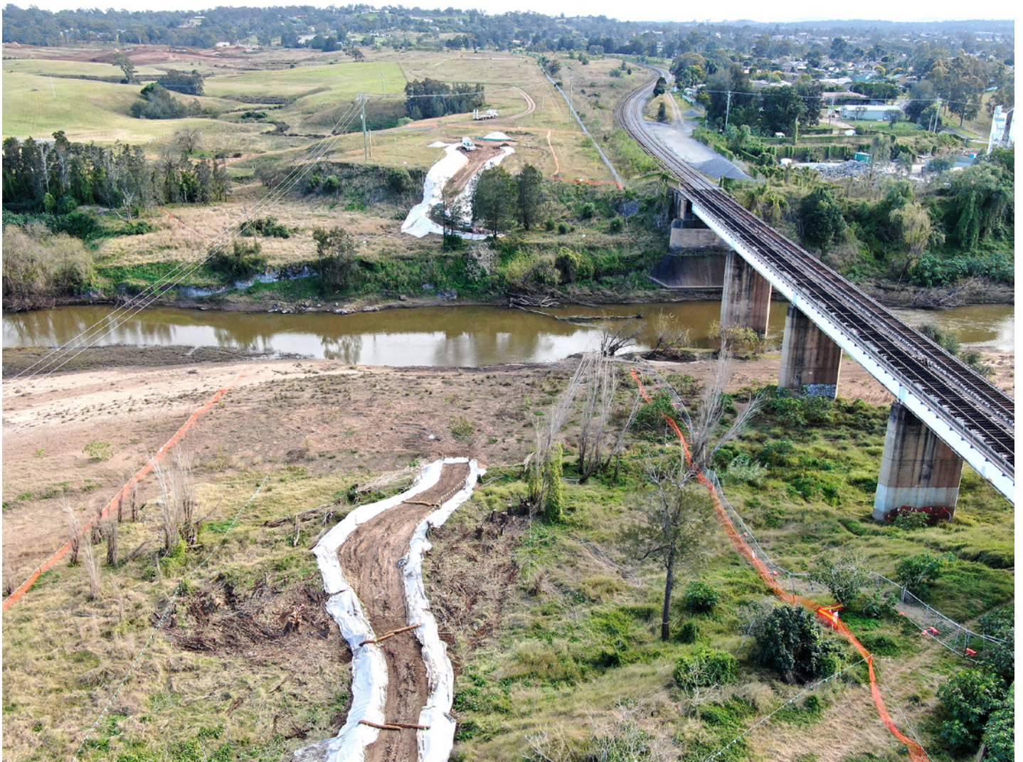
Earthworks for access tracks near the Hunter River
