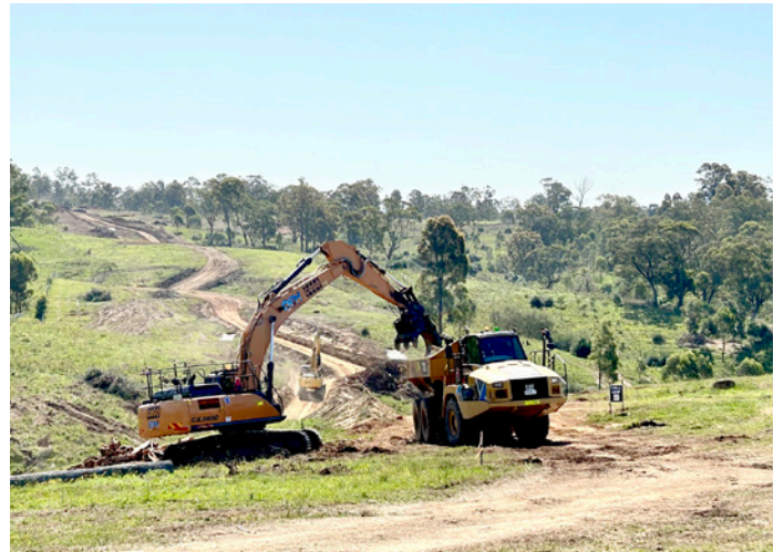
Earthworks on McDougalls Hill
